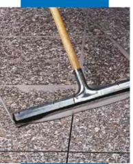
Grouting of pre-smoothened and glossed granite floor with rubber float
