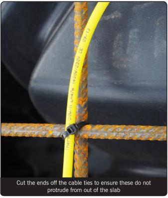
Once all the cable is laid out across the room, go back and tie off the cables at regular intervals (approx. 400mm intervals) to ensure cables are neat, held in place and protected. Do not have cables loose, dropping or too close to one another. Cut off the ends of the cable ties or ensure the tails are facing downwards so these do not protrude out of the slab. The heating cable is a single ended product so there is no additional cold tail to return.
