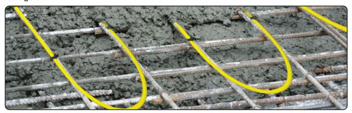
Roll up the cold tails and floor sensor cables that are protruding from your conduits so they are neat and out of the way of the contractors. We recommend that a qualified electrician is on site while the concrete is being poured to be constantly monitoring the resistance of the cable so any damage can be picked up immediately.
