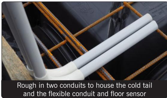
Rough in two conduits to house the cold tail and the flexible conduit and floor sensor
