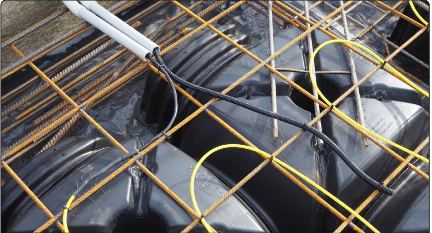
Feed the cold tail up the conduit and start running the heating cable from this position. Feed the flexible conduit for the floor sensor down the second conduit and install between two heating cables in a representative area of the floor.
