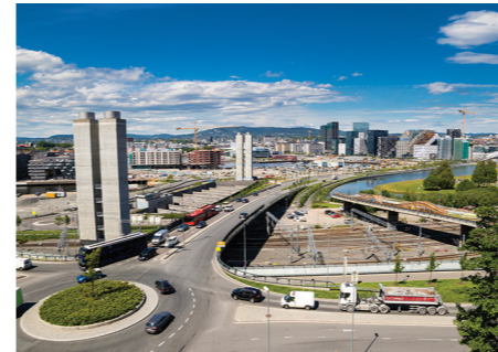
Bjørvika tunnel Oslo, Norway
